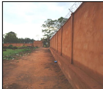
Newly completed DMGS perimeter wall
