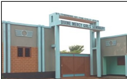
Newly completed DMGS entrance gate
